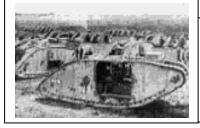
**Tanks** were used for the first time in the First World War. They were developed to cope with the conditions on the Western Front. The first tank was called 'Little Willie' and needed a crew of 3. Its maximum speed was 3mph and it could not cross trenches.
